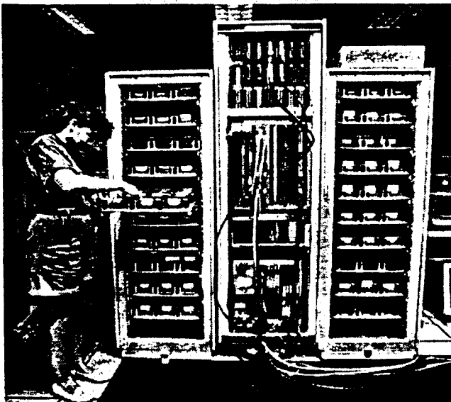
Figure 10: RAID-II Prototype Ann Drapeau is replacing a failed disk drive in the RAID-II storage server. The main equipment rack, containing the HIPPI boards, ATC disk controllers, VME links, and SUN host, is at the center. On either side are the racks of disk shelves. This configuration can hold up to 144 disk drives, 72 in each of the disk racks.
