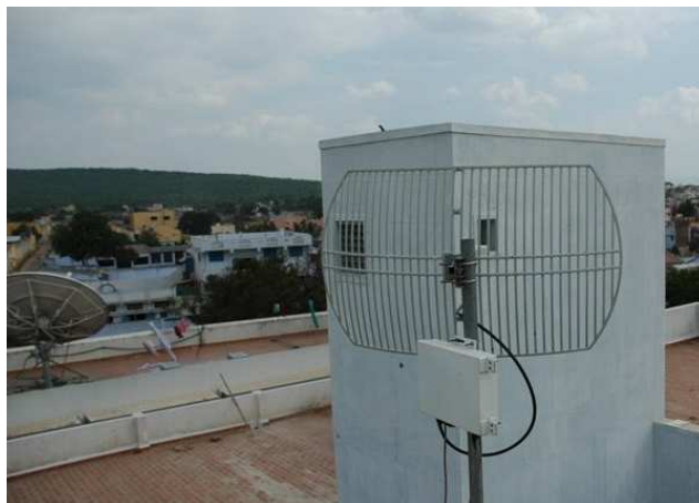
Figure 6.5: The Theni to Vijerani link in the Aravind network was completely obstructed by a newly constructed elevator shaft. This problem was not resolved until we visited Theni after 2 months.
