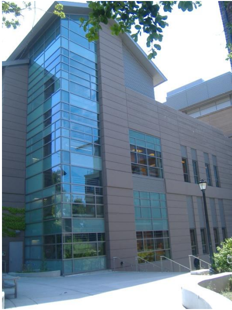
Fig. 33. Marvell NanoLab wing; the NW corner includes a clean stairwell between the two lab floors.
