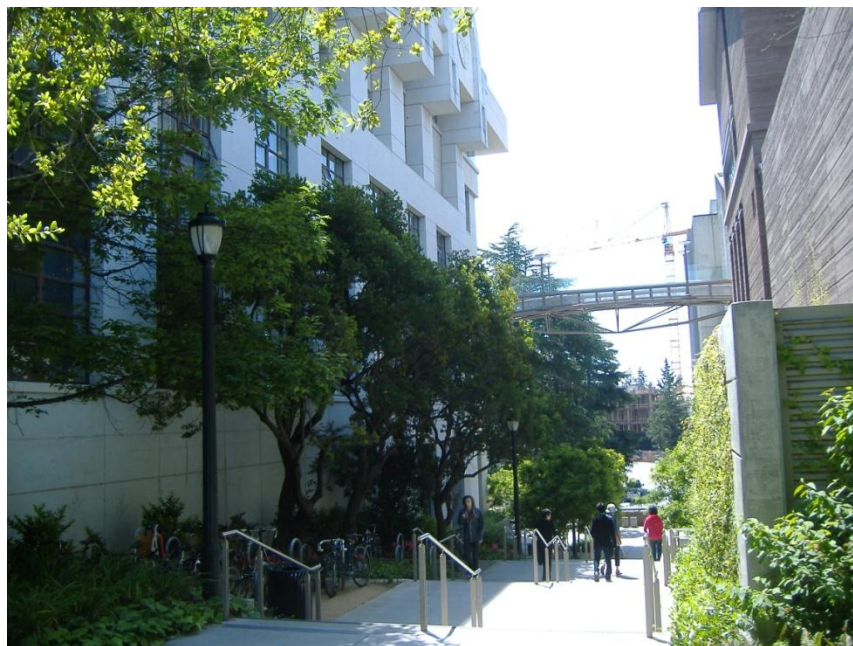
Fig. 38. The A. Richard Newton Bridge between Cory Hall (left) and SDH (right), viewed from Hearst Avenue.
