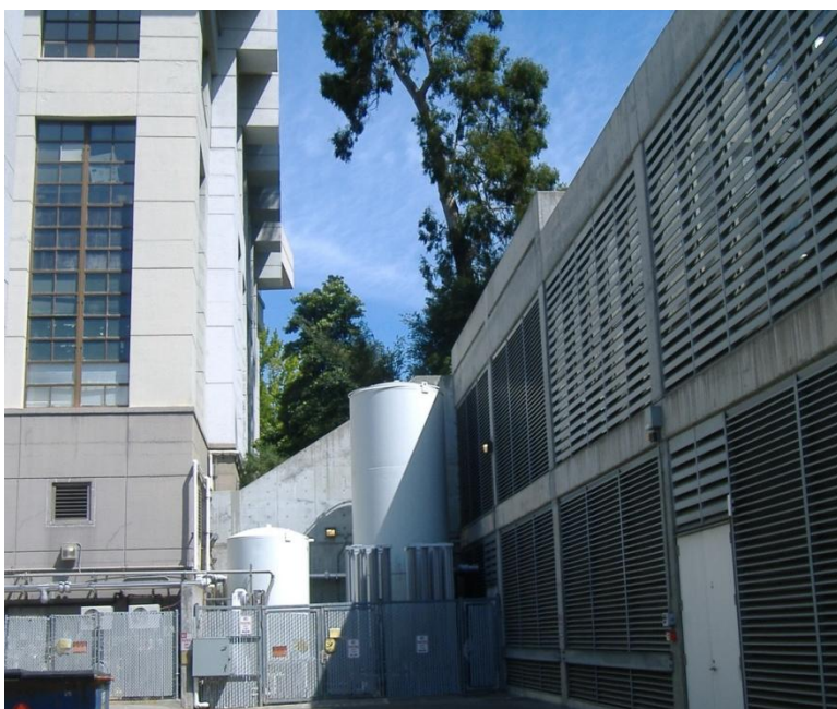
Fig. 28. Microlab LN vessels (3000 and 9000 gallons) and specialty gases service area, wedged between Cory Hall and HMMB's mechanical service building.
