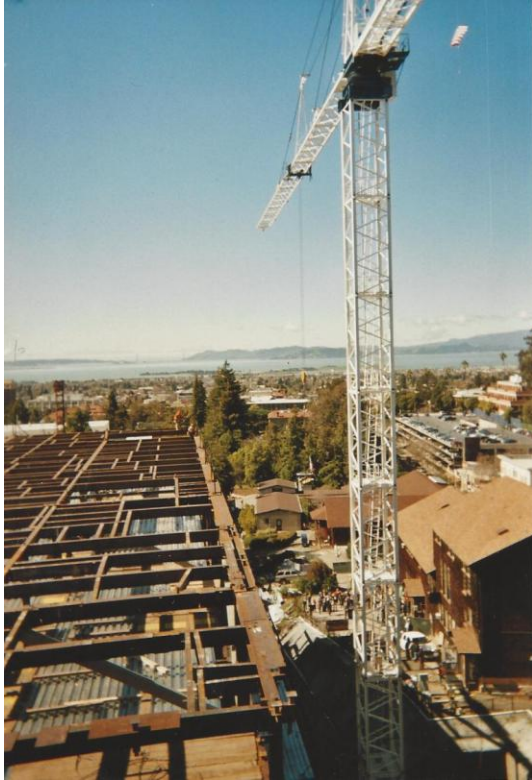
Fig. 30. (left) Construction of CITRIS Headquarters, seen from 406 Cory Hall (2007). (Before the structure blocked the Bay view.)
