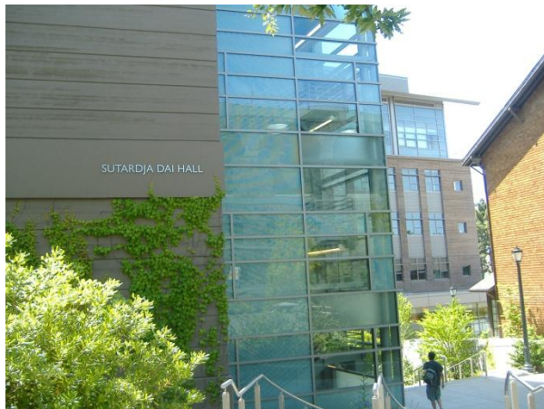
Fig. 35. Partial view of the NanoLab wing and the main part of Sutardja Dai Hall (SDH), as seen from Hearst Avenue.
