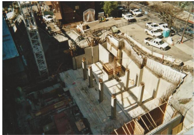
Fig. 31. (below) Sub-fab construction of the laboratory wing of the CITRIS building (2006).
