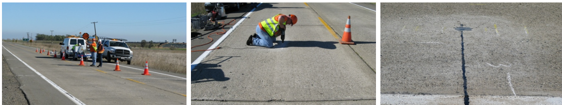
Figure 3.1: Sensor installation on Road 32A in Yolo County, California. ( left ) Single-lane road in each direction. ( middle ) Sensor location being drilled. ( right ) The output wire from the sensor is embedded in the road and connected to a road-side NI DAQ box for data collection.
