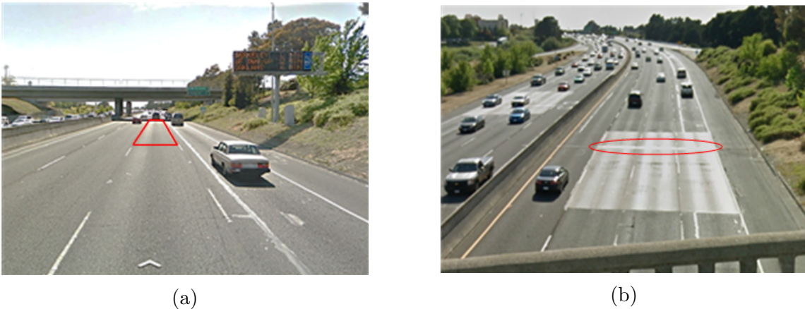
Figure 3.7: Pinole site. (a) Sensors installed in lane 2, location outlined in red. The AP and camera are installed on the road-side pole. A conventional WIM station is located right after the overpass. (b) View of the WIM station from the overpass.
