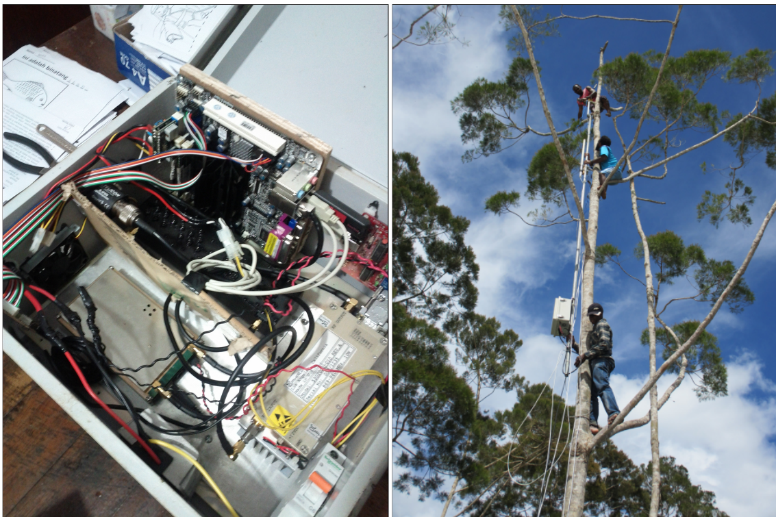
Figure 6.1: Our Base Station and its installation.
