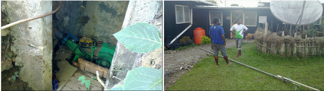
Figure 5.2: The existing infrastructure: Hydroelectric power and VSAT.
