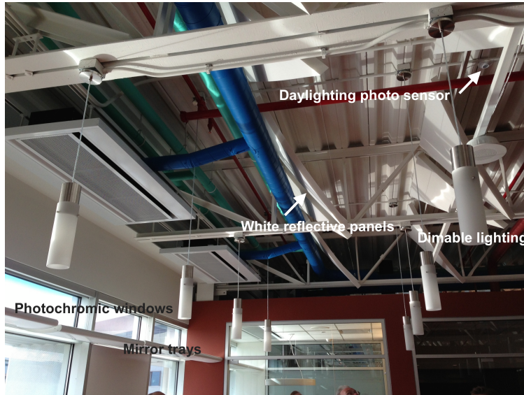
Figure 2.2: A building interior at the National Renewable Resources Laboratory exhibiting many active and passive features designed for daylighting.
