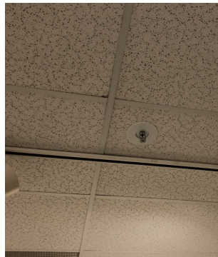
Figure 3.2.: Fire sprinkler asset training image example
