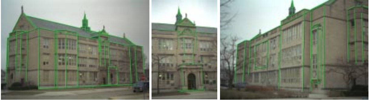
Figure 9: Three of the twelve photographs used to reconstruct a high school building. The green lines indicate the edges the user has marked.
