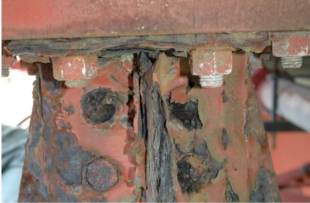
Figure 4.3. Severity of rusting of the bridge can be seen. Rusting not only threatens the bridge, but also was a hazard to the monitoring system, see Figure 4.1
