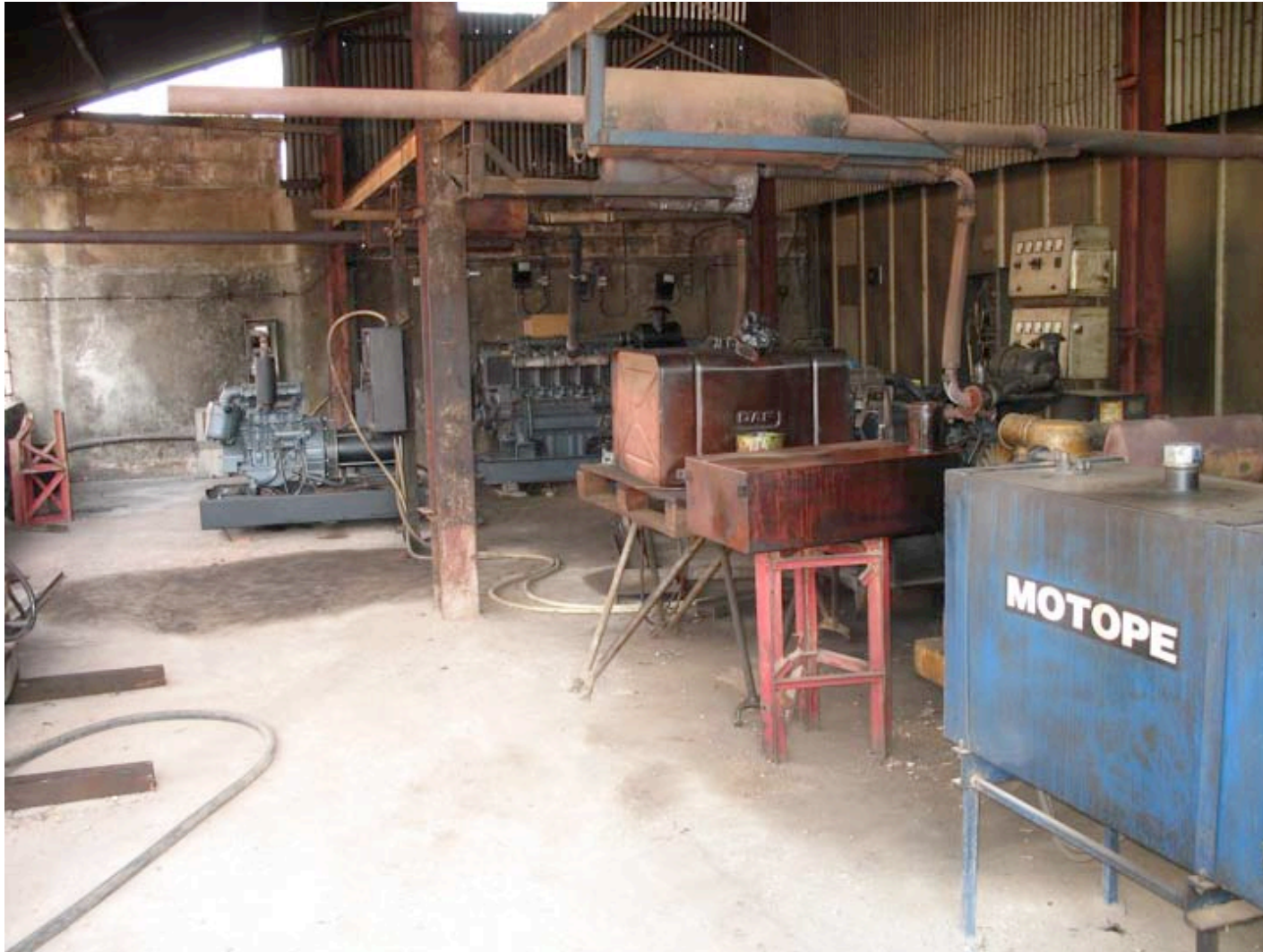
Figure 1.4: A building housing generators for an ISP in Guinea Bissau. The closest generator was poorly tuned and exhausted into the room, causing dangerous levels of carbon monoxide to accumulate in the work area.
